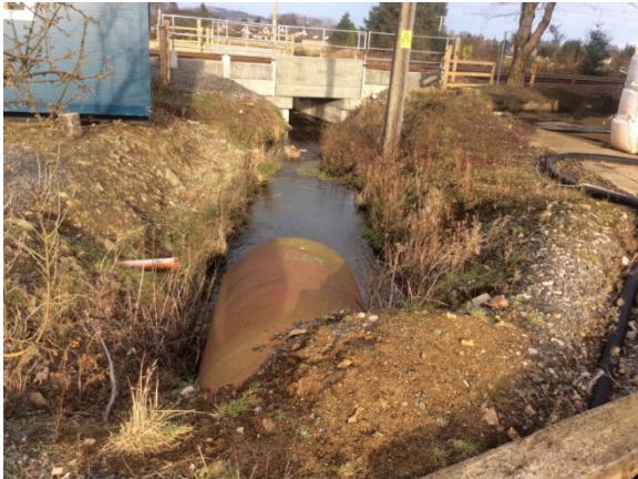
Upstream view of pipe
