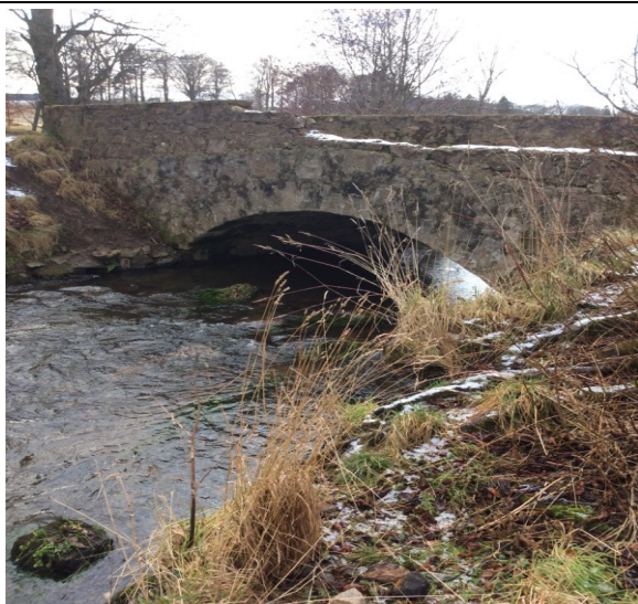
Downstream view of bridge
