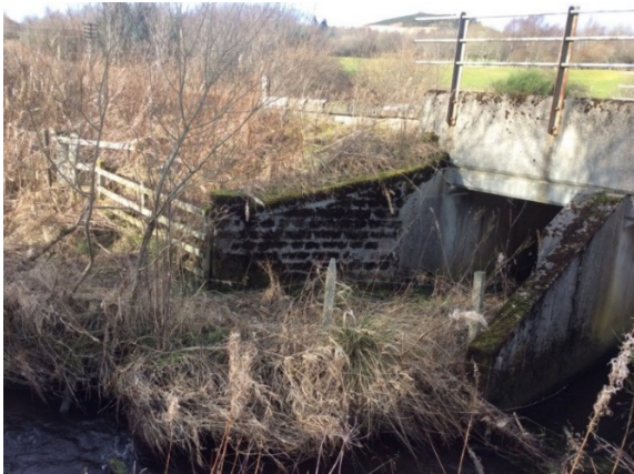
Upstream view of left abutment
