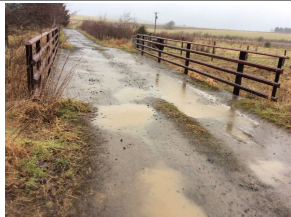
View of bridge
