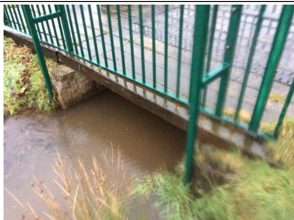
Downstream view of bridge
