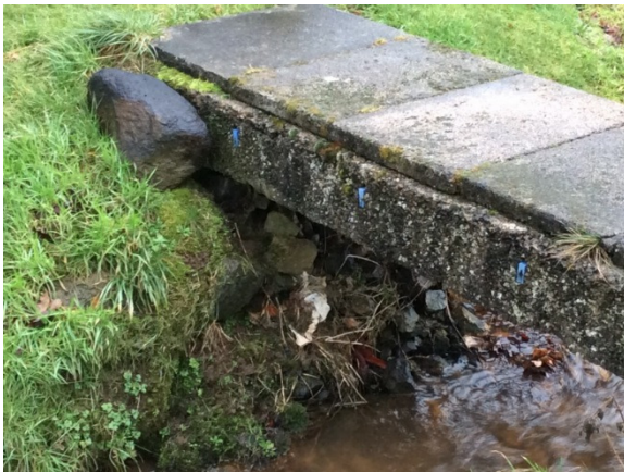
Closer view of bridge from downstream
