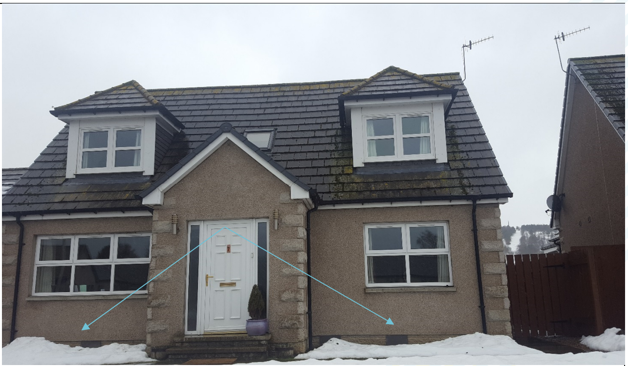
Figure 9-4: Property Level Protection of 7 Mill Road
