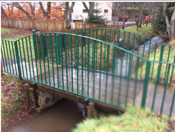
Upstream view of bridge
