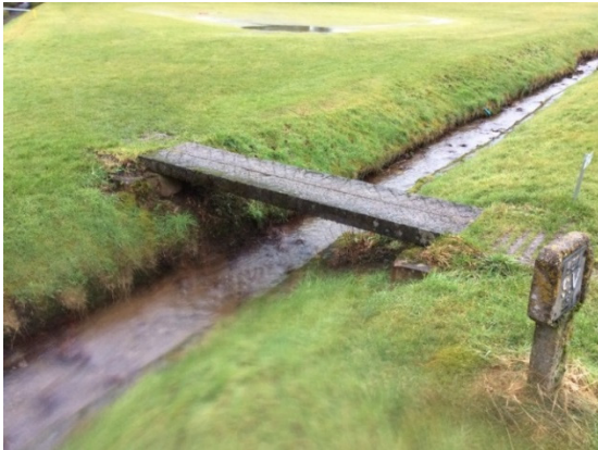
Downstream view of bridge
