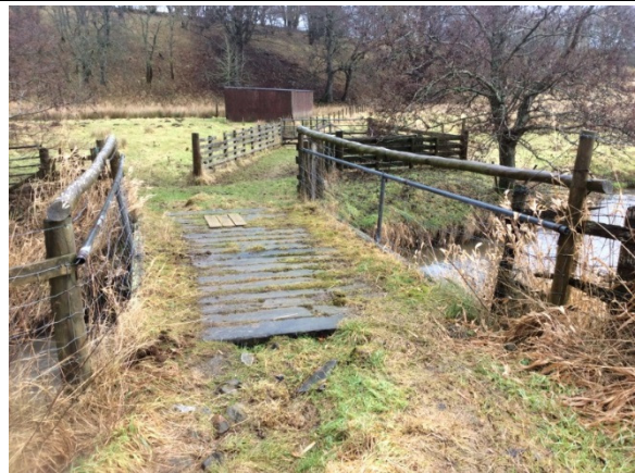
View of bridge
