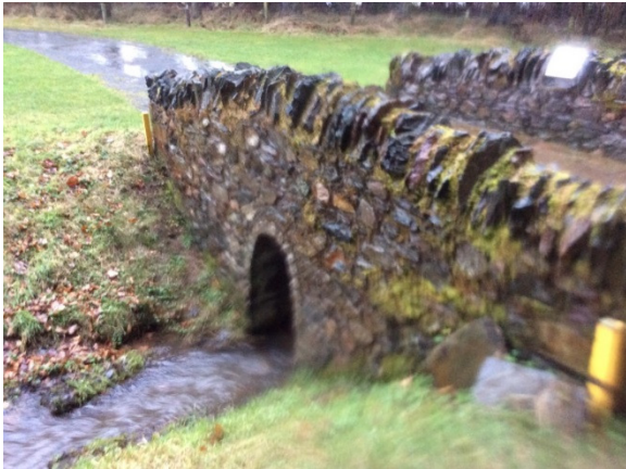
Upstream view of bridge
