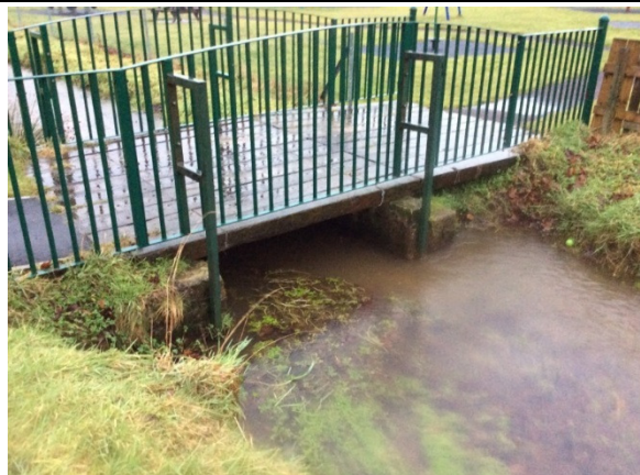
Upstream view of bridge
