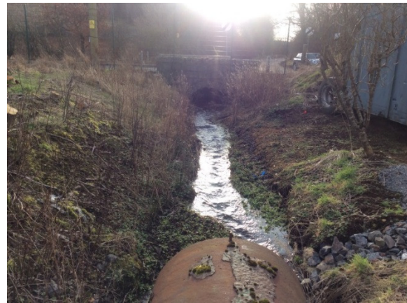
Upstream side of culvert
