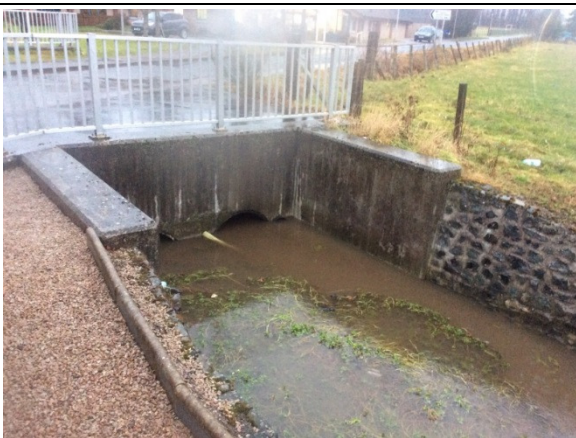
Downstream view of bridge
