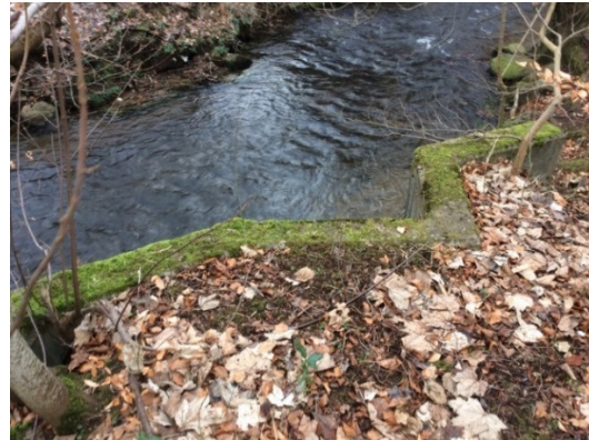
View of wall from above looking downstream
