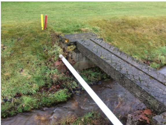
Downstream view of bridge
