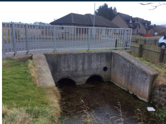
Upstream view of bridge
