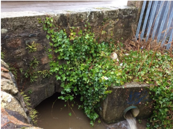
Downstream view of bridge
