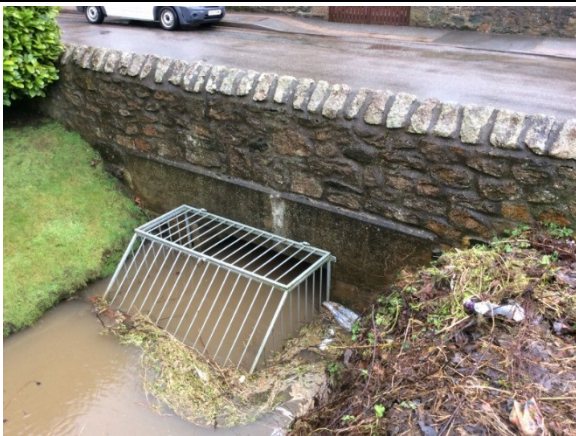
Upstream view of bridge
