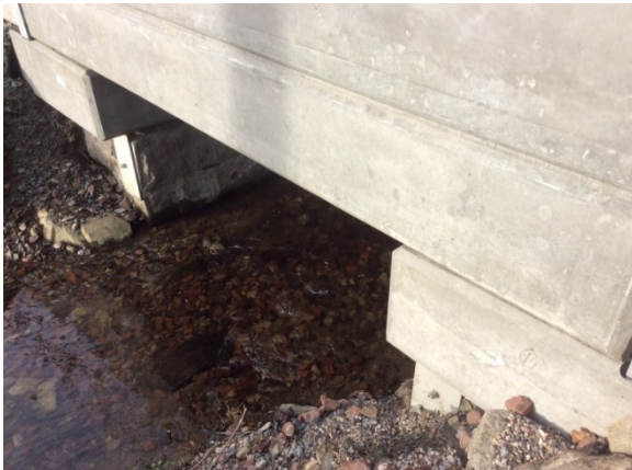
Downstream view of abutments
