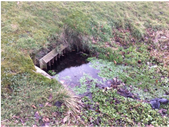
Culvert outlet with screen
