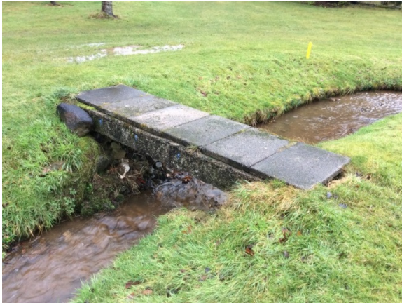
Downstream view of bridge
