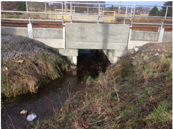
Downstream view of bridge
