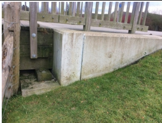
Right abutment and fixings
