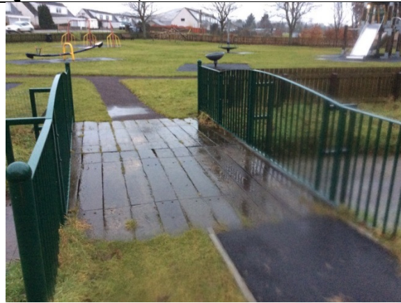
View of bridge
