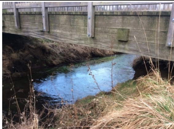
Bridge deck, upstream view
