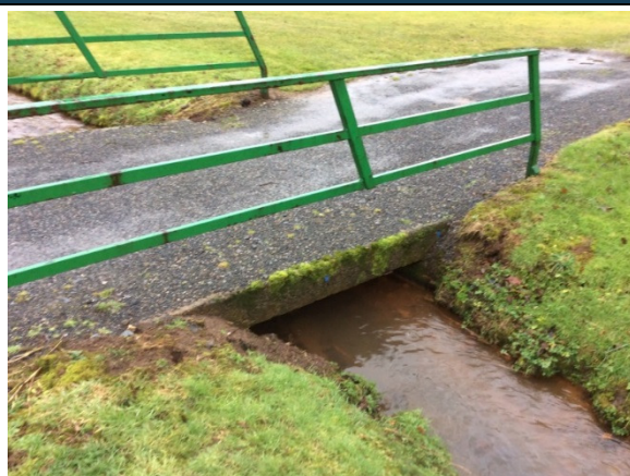
Upstream view of bridge
