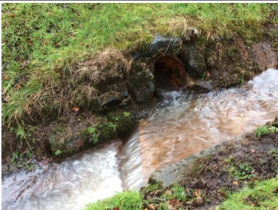
Downstream view of weir
