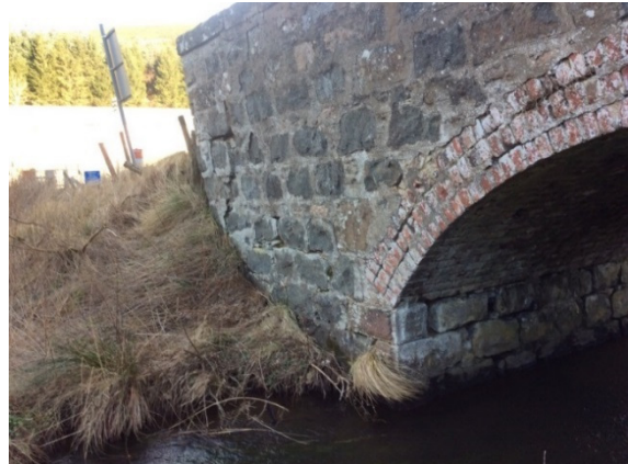
Upstream view - Left abutment
