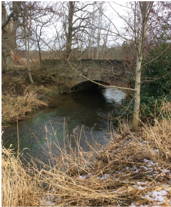
Upstream view of bridge
