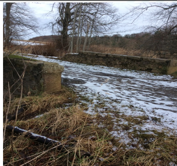
View of bridge
