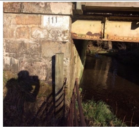
Upstream view – Left abutment
