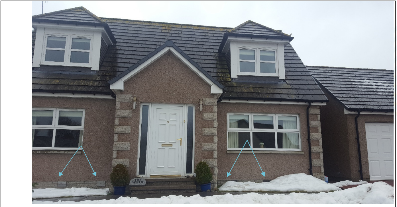
Figure 9-5: Property Level Protection of 9 Mill Road
