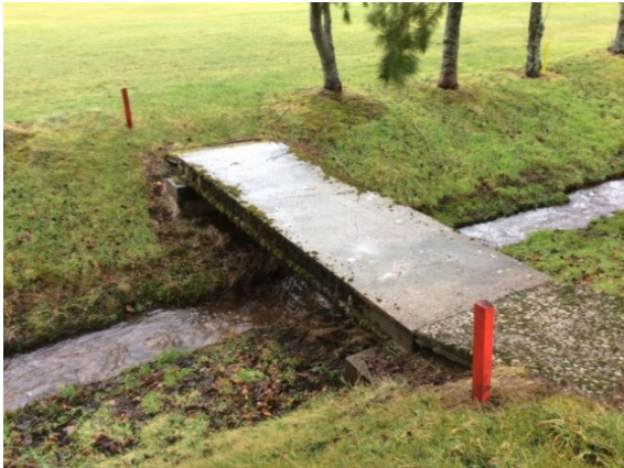
Downstream view of bridge
