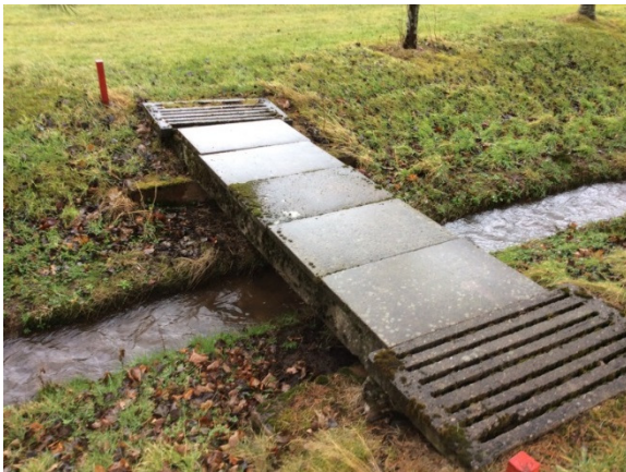
Downstream view of bridge
