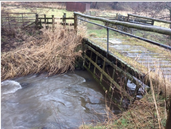
Downstream view of bridge
