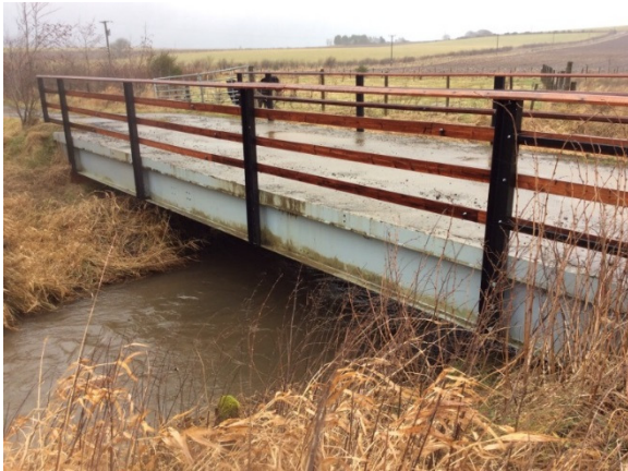
Upstream view of bridge
