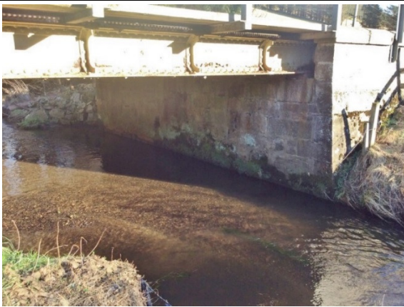
Upstream View – Right abutment
