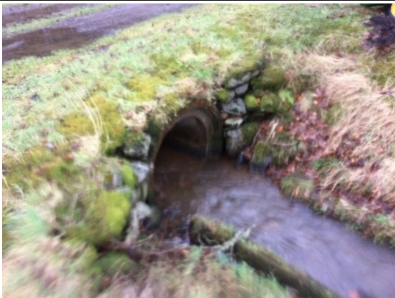
Upstream view of culvert
