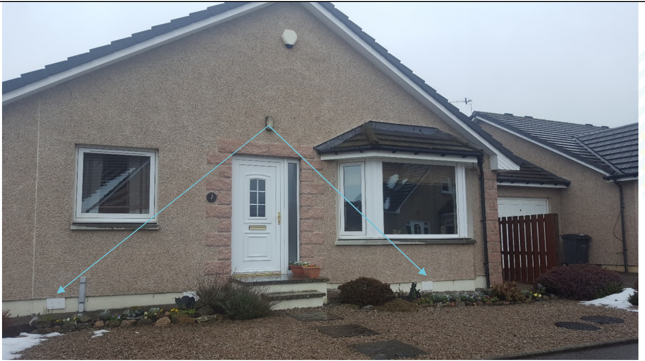
Figure 9-3: Property Level Protection of 7 Old Mart Avenue
