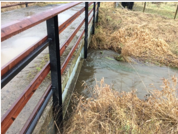
Downstream view of bridge
