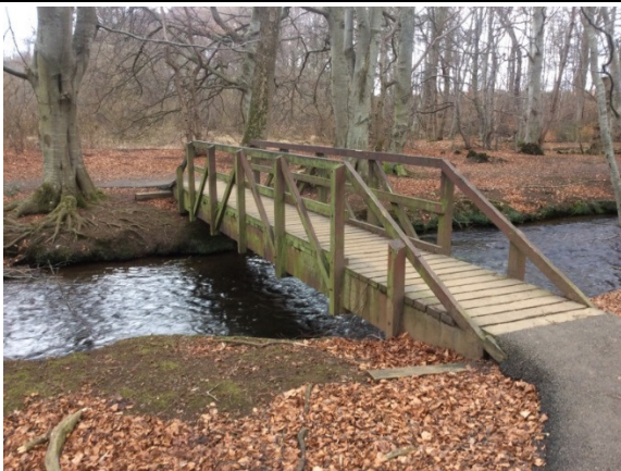
Upstream view of bridge
