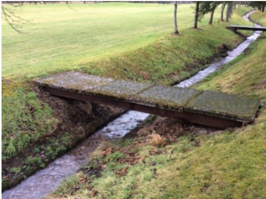
Downstream view of bridge
