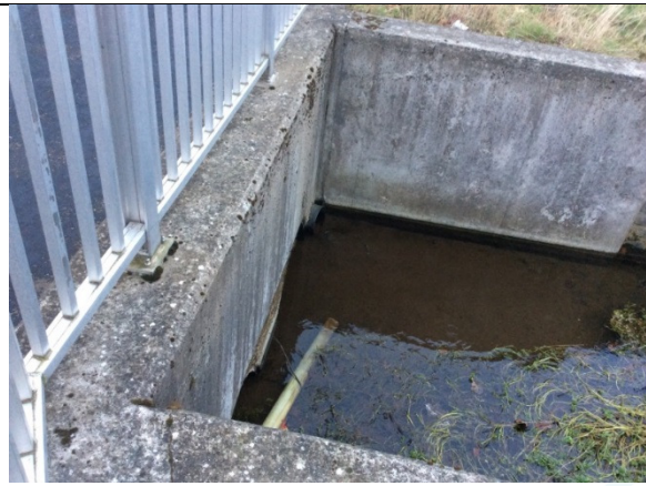
Downstream view of concrete walls
