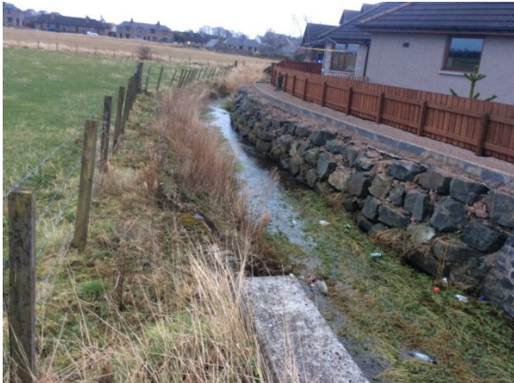
Upstream view of wall
