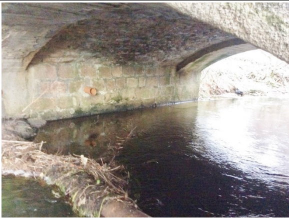
Downstream view of soffit
