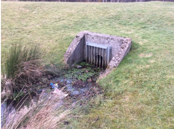
Inlet pipe and headwall with bar screen (Sinks)
