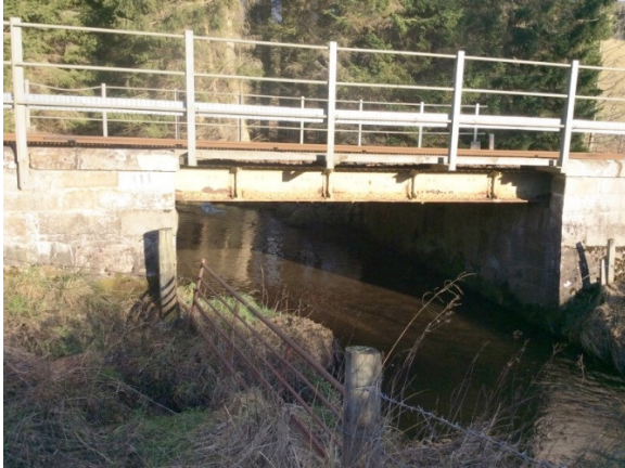
Upstream view of bridge
