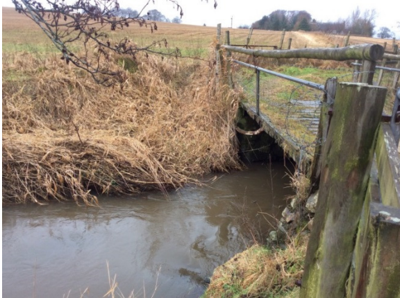
Upstream view of bridge
